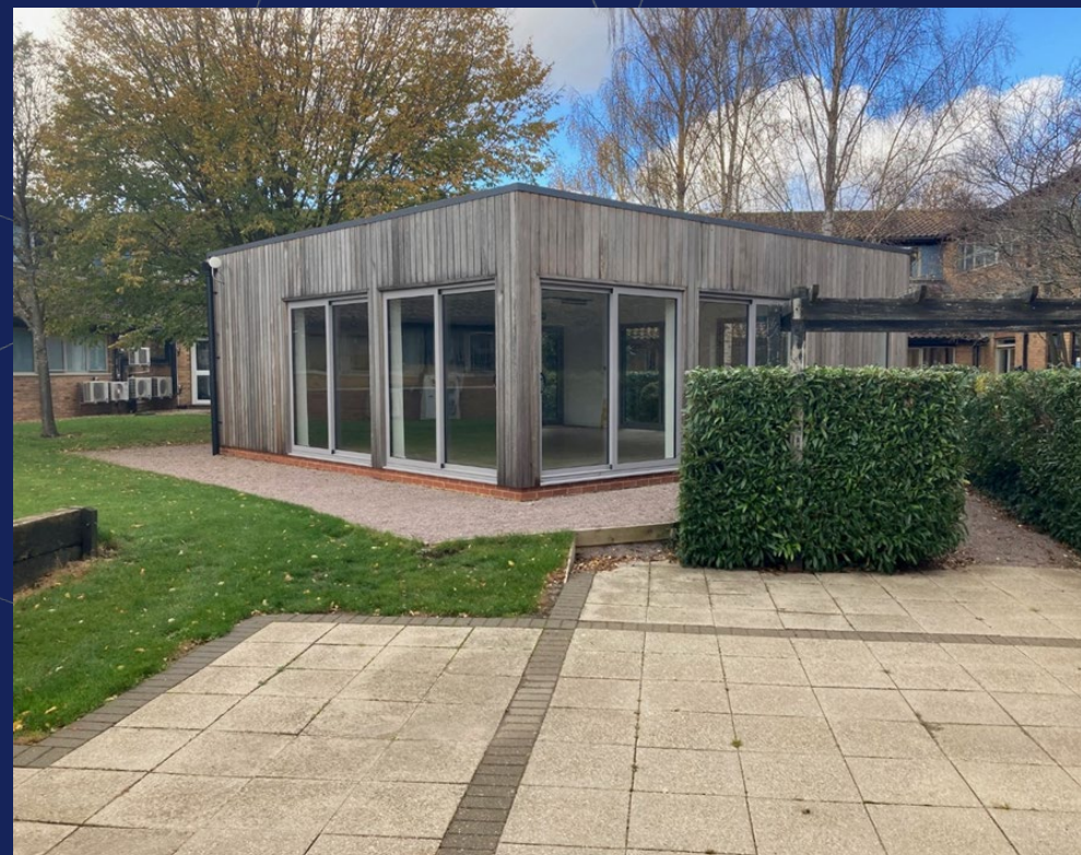
Block H, Garden Room
