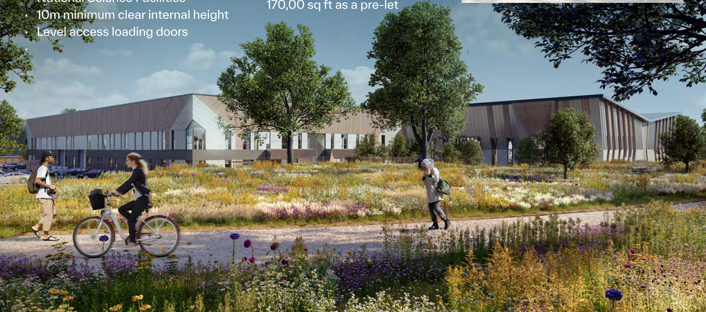
TF1 and TF2 having the zinc and timber cladding finalised.
