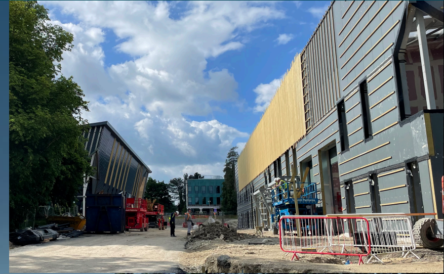
TF1 and TF2 having the zinc and timber cladding finalised.
