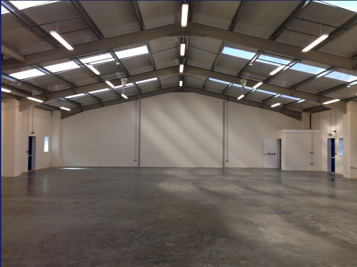
Warehouse prior to occupation
