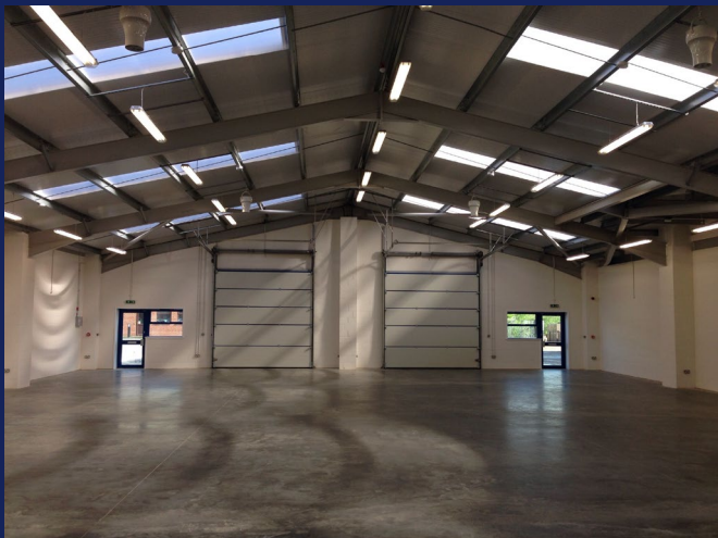
Warehouse prior to occupation
